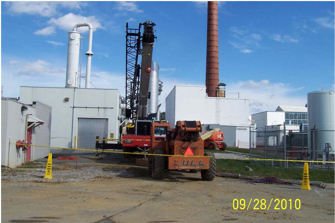
Crane used to lift stacks.
