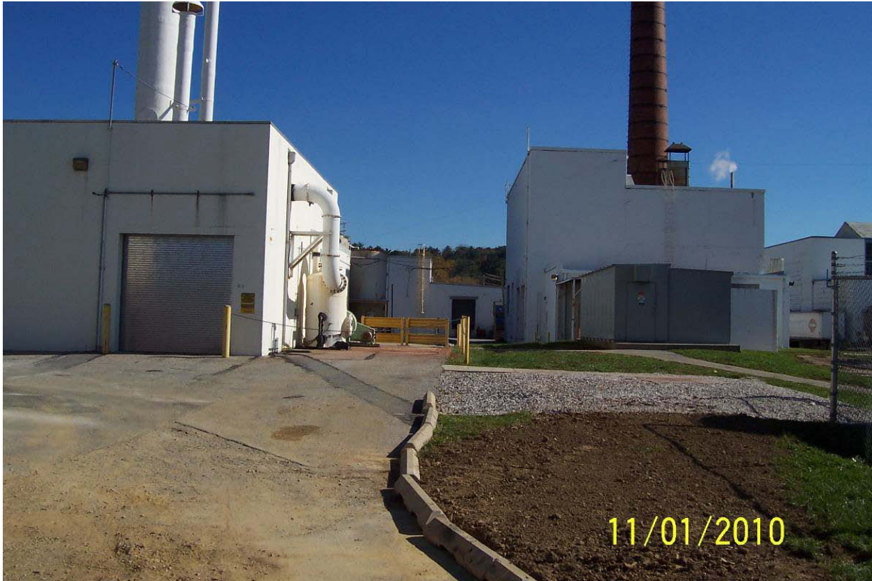
Looking east at the TFO pad after the TFO and hydrogen storage area were removed.
