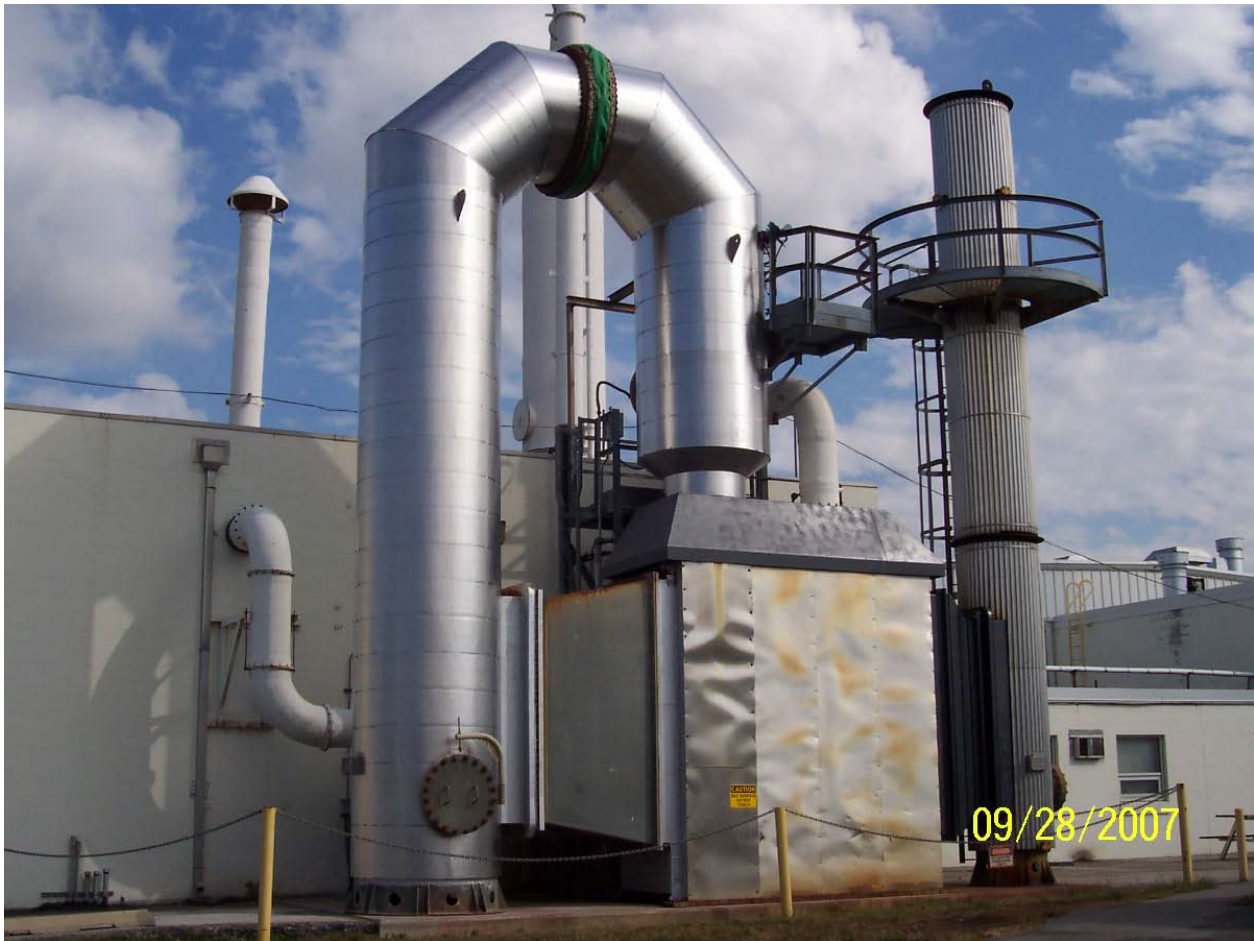
TFO before demolition.
