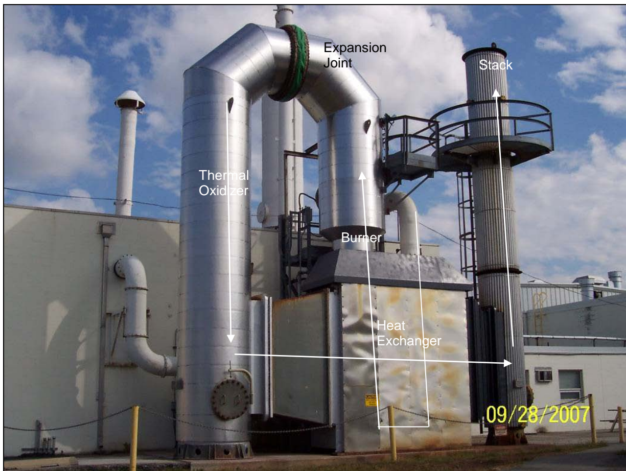
Figure 1. Photo of Thermal Fume Oxidizer before demolition (arrows show direction of off-gas flow).
