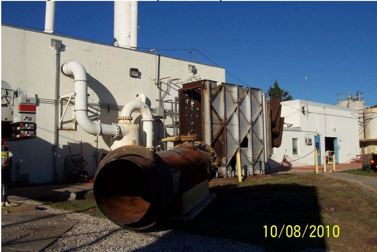
The eastern stack is on the ground for demolition.
