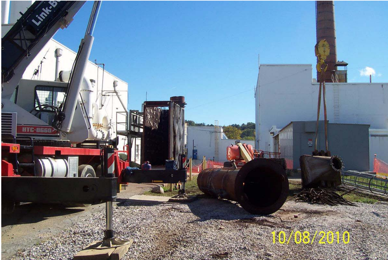
TFO looking east. Both stacks, the recuperator, and the platform was removed.
